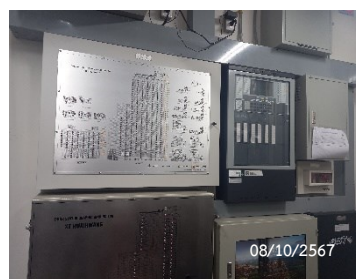
Graphic Annunciator Fire Alarm System
